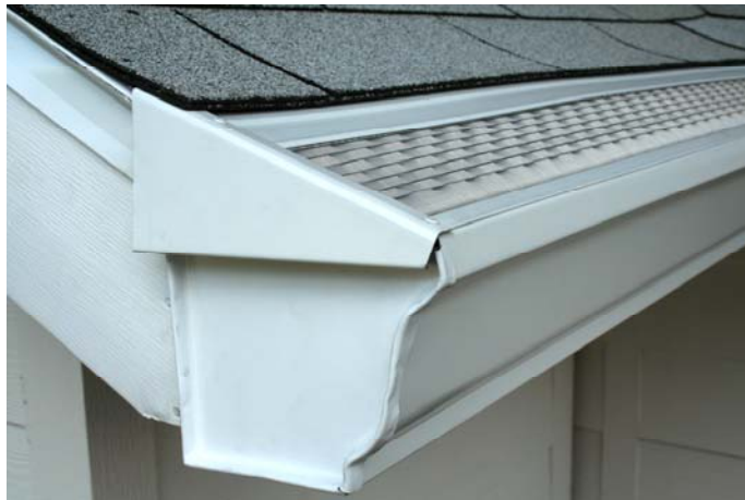
Field fabricate end cap cover
