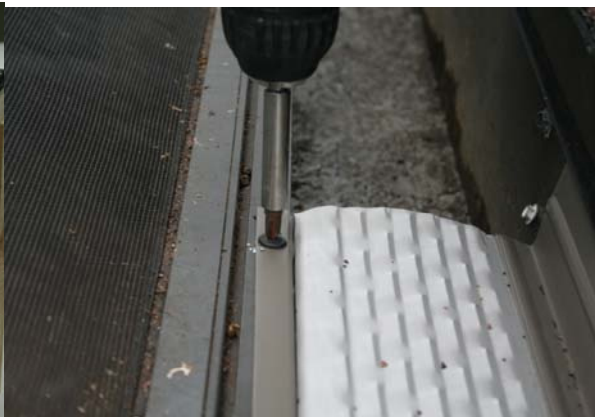
Secure in place to the gutter lip
