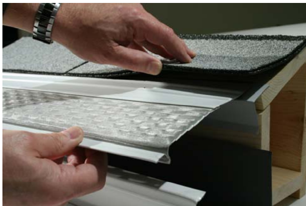
Installed beneath 1 st shingle
